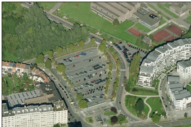
Figure 12 Zone du parking Rodebeek
